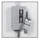
When preparing to remove or install a motor, put safety first. Wear appropriate personal protective equipment (PPE). Follow applicable electrical codes for wiring, disconnect and emergency stop requirements. Lock out and tag out all potential energy sources before working on the motor. Use safe lifting methods appropriate to the motor's size and weight.
